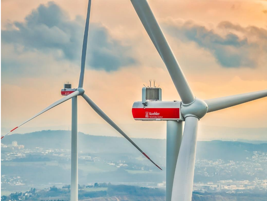
Figure: The construction of its wind farm in Wetzlar-Blasbach/Germany represented a milestone for the Koehler Group and is an important part of the company's ambitious climate strategy. Source: Koehler Group
